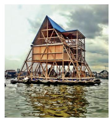
Makoko Floating School, prototype structure for the coastal water community of Makoko, Nigeria. The triangular A-frame is an ideal shape for a floating object due to its low center of gravity, which provides stability even in extreme weather conditions. Green buildings play a significant role in building resilience against future climate change and natural disasters. © *NLÉ Architects*
